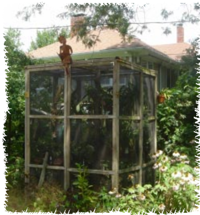
Shadehouse at the Parkison's House
